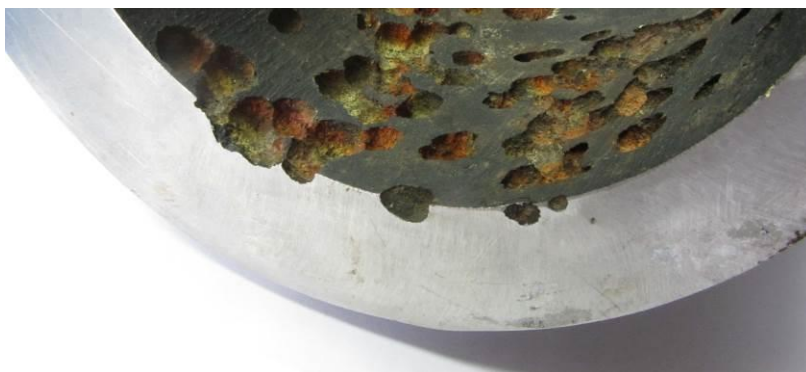
Large Corrosion Pits.
