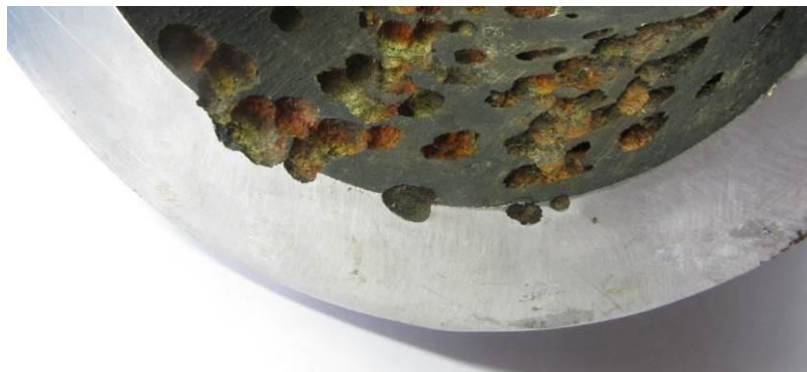
Large Corrosion Pits.
